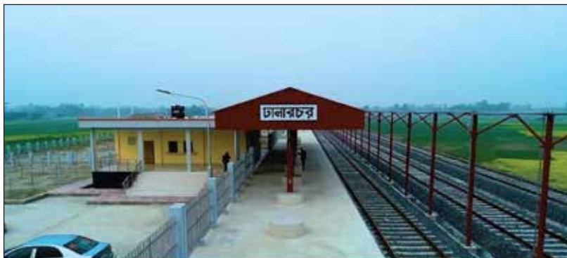
Newly built Dhalarchar Railway Station under the project 'Construction of a New Railway Line from Ishurdi to Dhalarchar via Pabna'.
